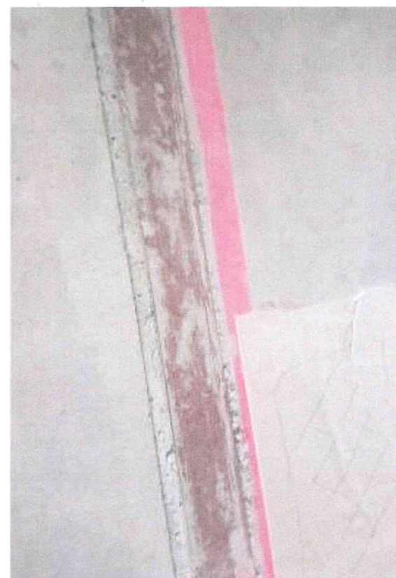
COVER PLATE OVER SEISMIC GAP BETWEEN LAB (HA26) AND AAU (HA34)
