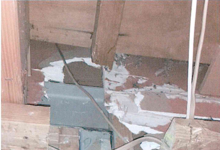
STEEL BEAM AND POST ALONG CORRIDOR (PHOTO TAKEN FROM ADJACENT BUILDING)
