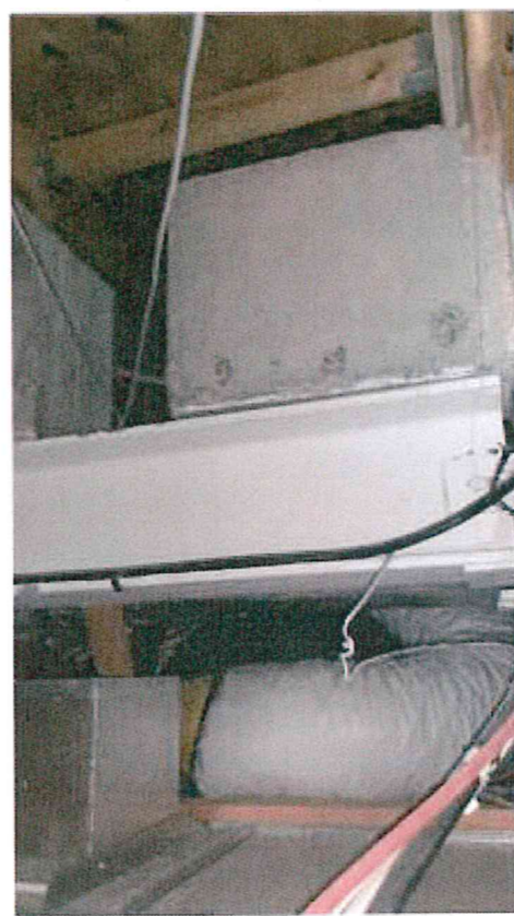
SEISMIC GAP BETWEEN LAB (HA26) AND AAU (HA34)
