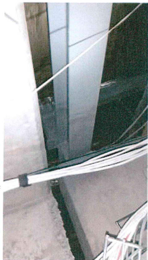
SEISMIC GAP BETWEEN LAB (HA26) AND ED (HA25)
