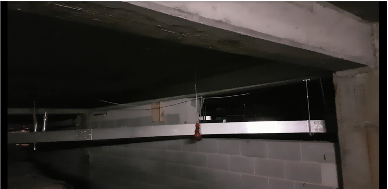
Figure 40: Wall No. 5 (left) and 6 (right)
