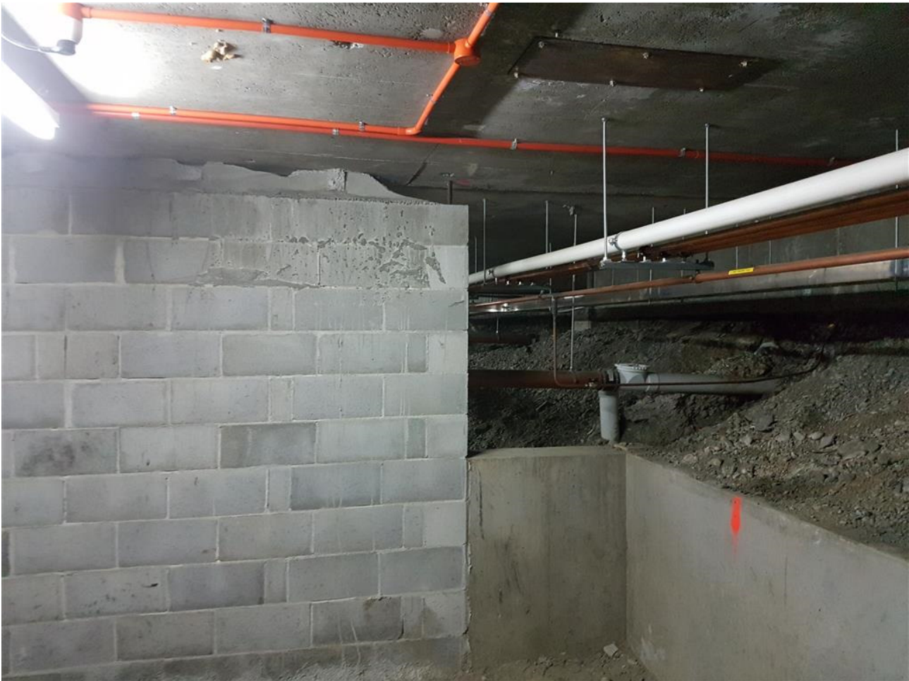
Figure 20: Example of RCM wall with incomplete infill and lack of dowel action at top.
