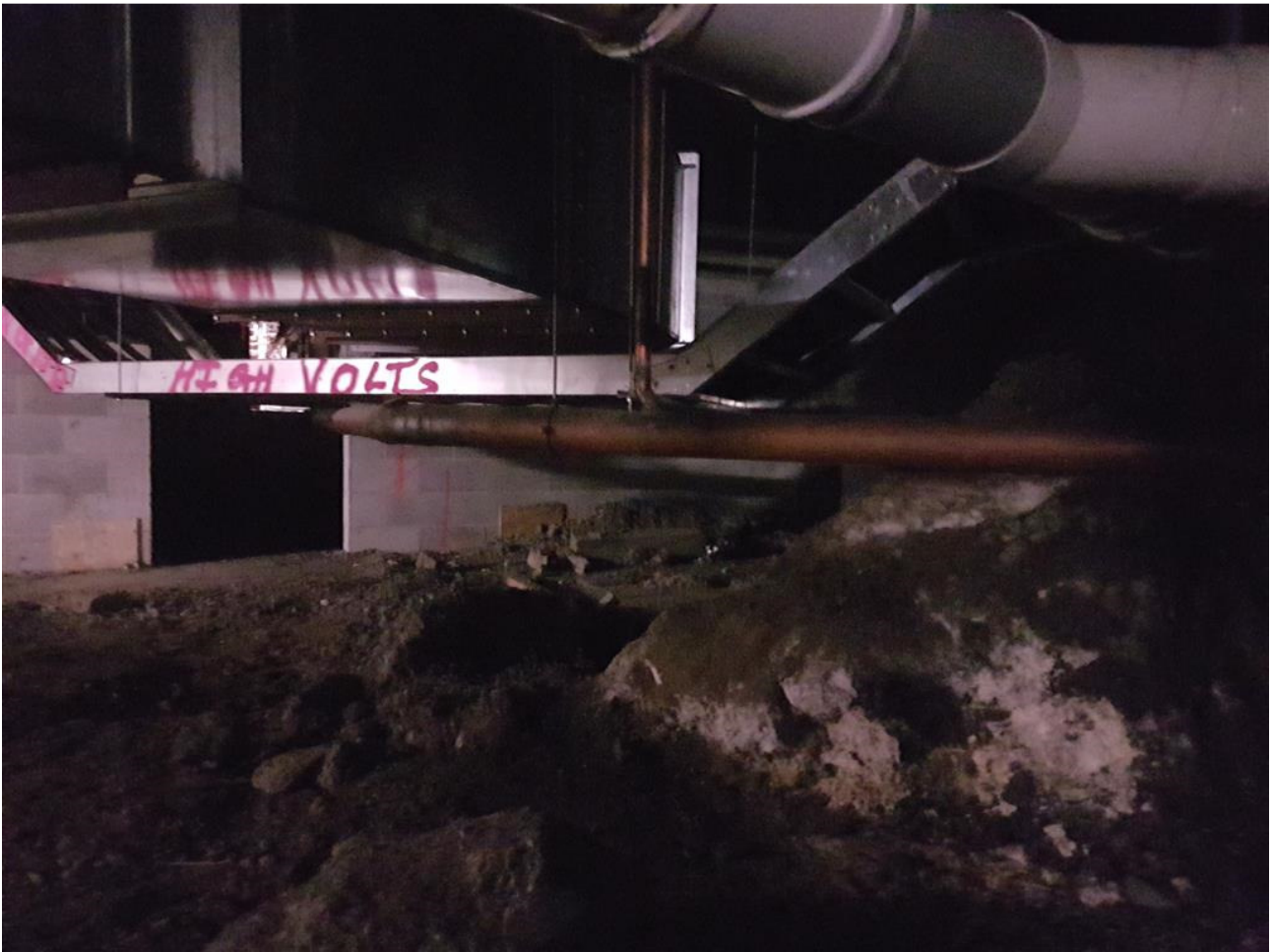
Figure 53: Wall #21 – Uncomplete height on left, lack of dowels on right
