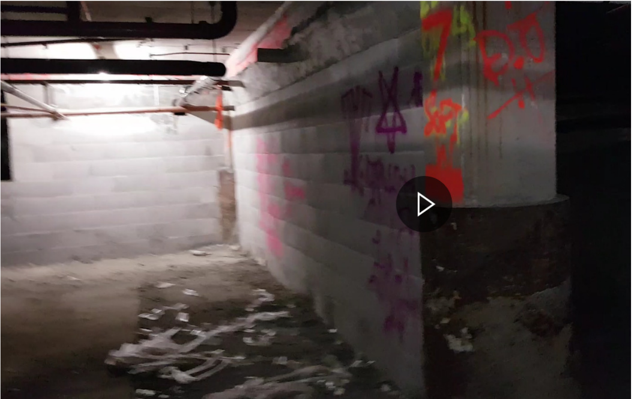
Figure 52: Wall #20 (left) and #5 (right)
