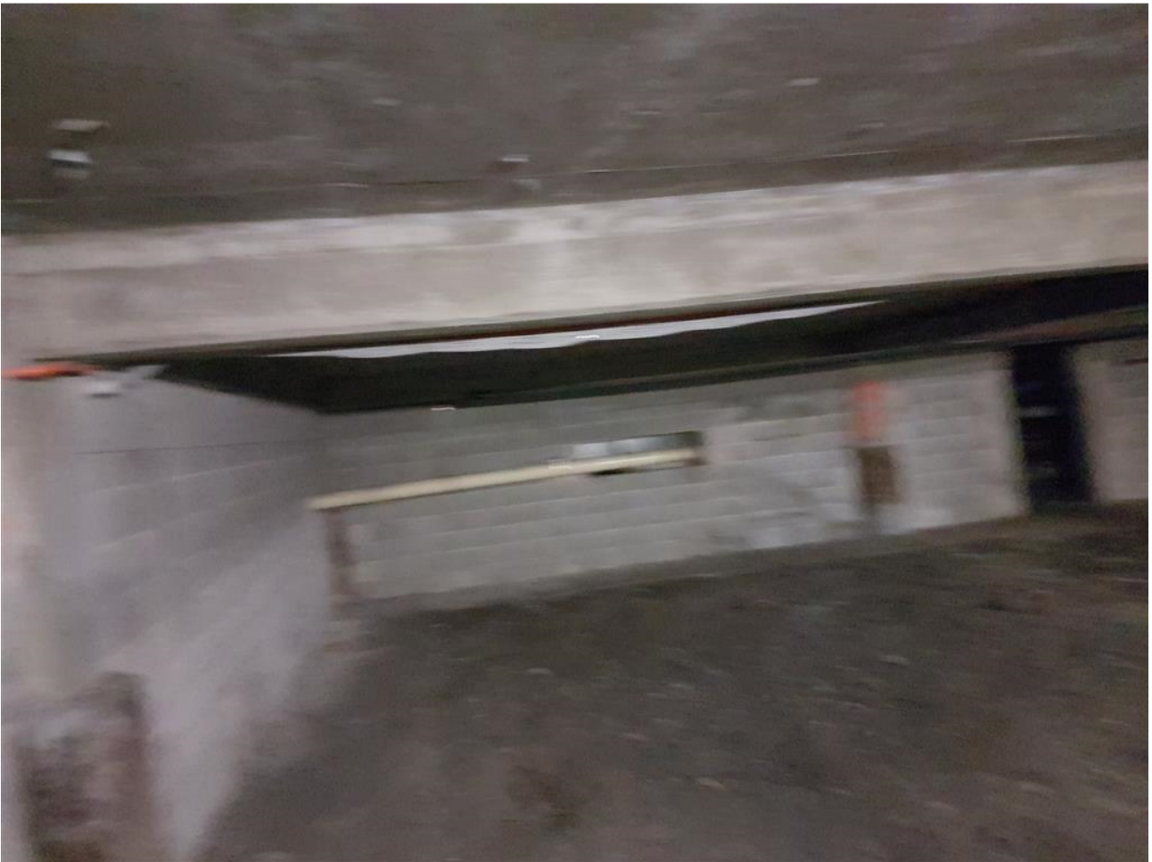
Figure 57: Wall #25 – With Opening
